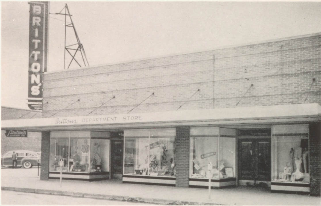
LEBANON'S HOME-OWNED DEPARTMENT STORE
