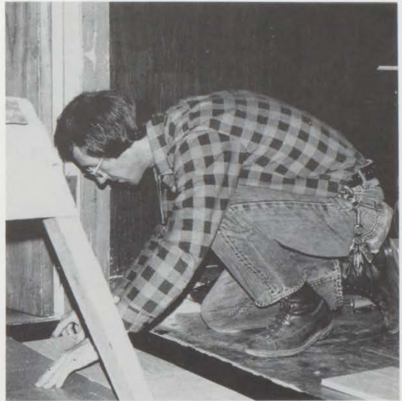
Mr. Ron Peters replaces worn tiles on the auditorium stage.
