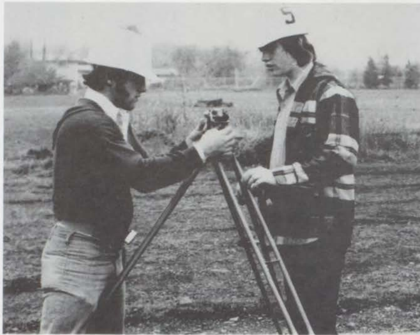
Jimmy Matlock and Bryon Patterson set the sights for building construction.
