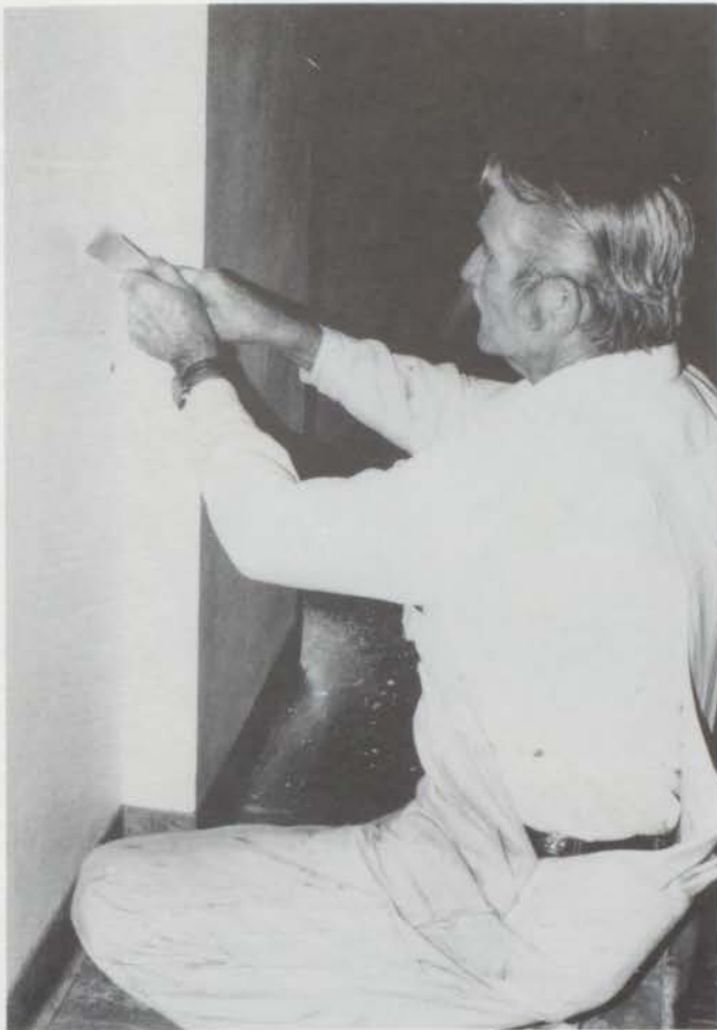
Mr. Joe Stewart scrapes plaster off the wall to prepare it for the new wall murals.
